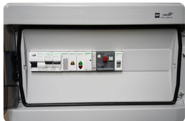
Control box (with electric shock protection in the form of a RCD circuit breaker and a pump motor switch). Additionally equipped with a light and sound alarm, and mode switch. 18-module casing with IP 65 rating. three float switches are connected to the box.
