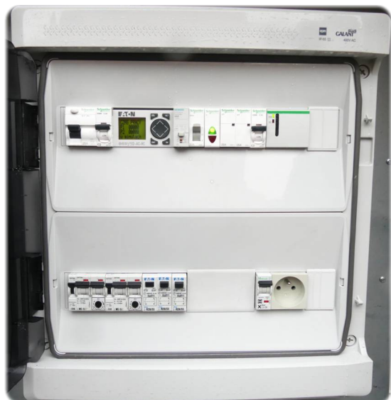
Control box for 2 single-phase pumps (with electric shock protection in form of RCD and pump motor circuit breaker for both pumps). Equipped with a warning light, operating mode switch, PLC controller with information display and GSM module (remote notification of malfunction), three float switches enclosed in a 36-module housing with IP 65 rating
