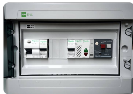
Protection and alarm box (with shock protection in the form of a RCD circuit breaker and a pump motor switch). Additionally, it is equipped with a light and sound alarm. 12-module casing with IP 65 rating. single float switch is connected to the device.
