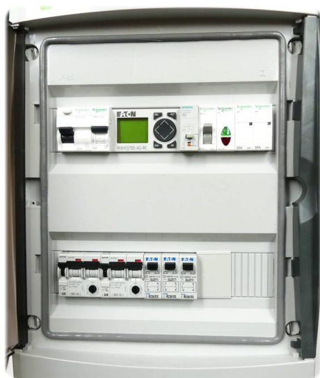
Control box for 2 single-phase pumps (with electric shock protection in form of RCD and pump motor circuit breaker for both pumps). Equipped with a warning light, operating mode switch, PLC controller with information display, three float switches enclosed in a 24-module housing with IP 65 rating
