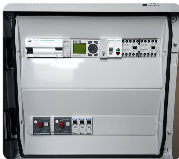
Control box for 2 three-phase pumps (with electric shock protection in form of RCD and pump motor circuit breaker for both pumps). Equipped with a warning light, operating mode switch, Phase controller (loss and phase order) PLC controller with information display, three float switches enclosed in a 36-module housing with IP 65 rating
